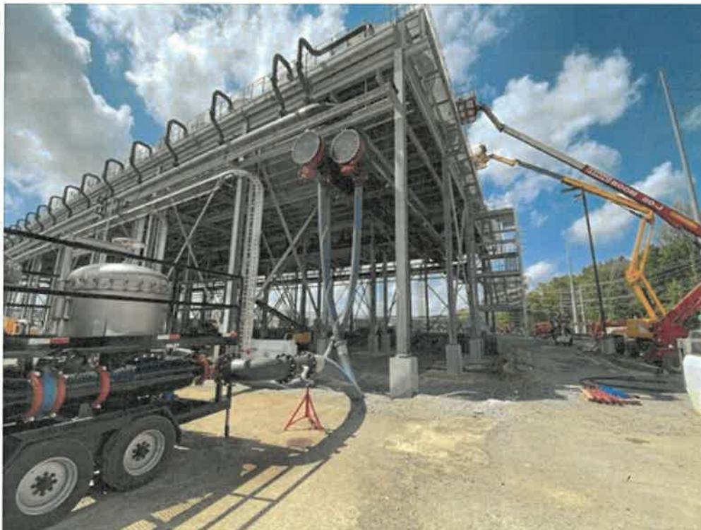
Photo 4-Looking north from the southeast corner of the closed loop dry cooling tower structure.
