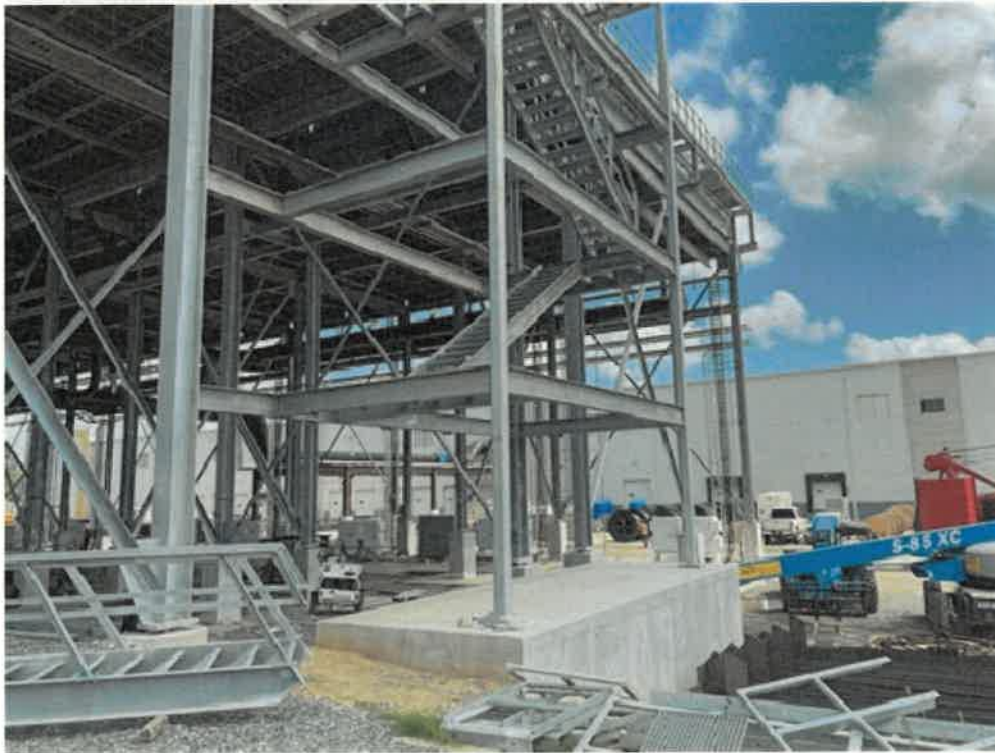
Photo 6-Looking southeast at north side of building from northwest corner of cooling tower.
