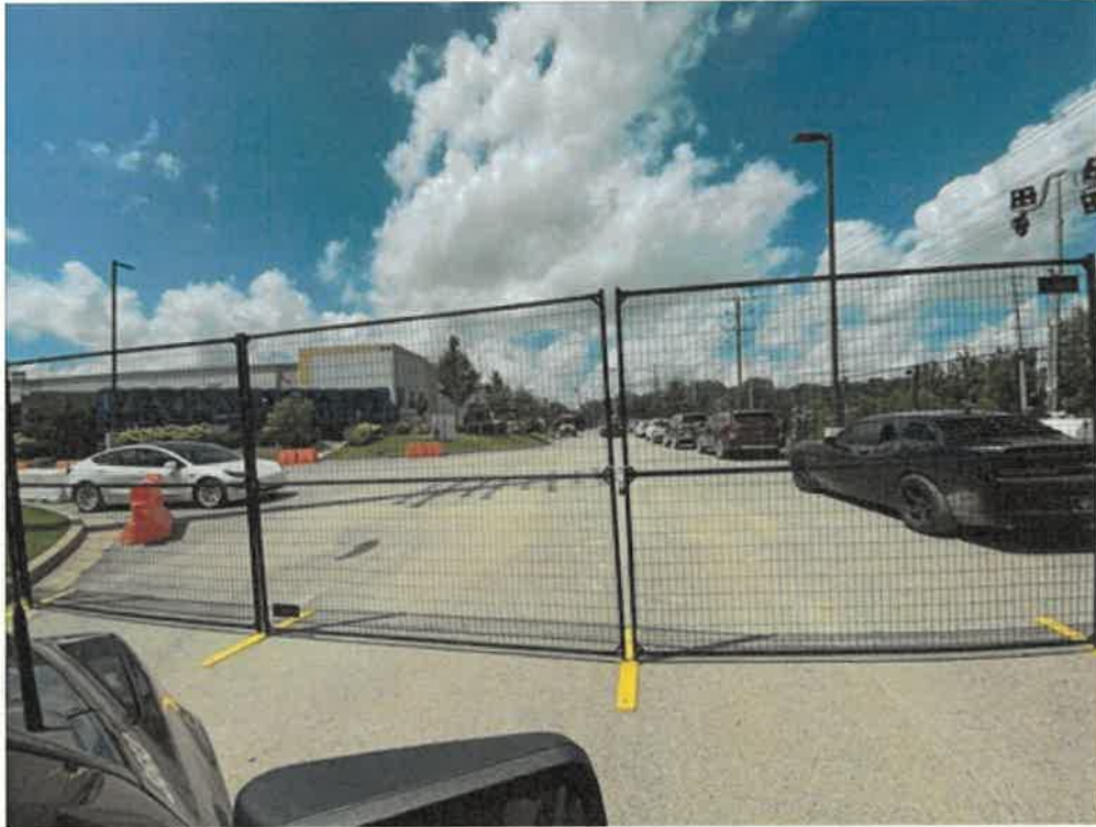
Photo 1-The site entrances along Stateline Road have been locked shut with temporary fence panels. Note mobile cooling units around building.
