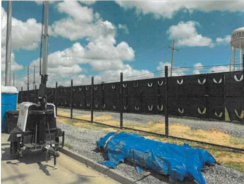
Photo 9-Section of new fencing in front of temporary fence panels with black privacy screening. This is along the south perimeter.
