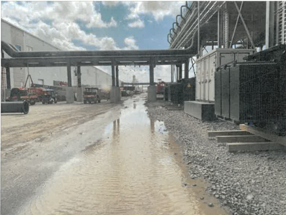
Photo 8-Looking west at existing piping to cooling tower structure. Horizontal structure in background is fiber bridge, with TVA Southaven visible in far background.
