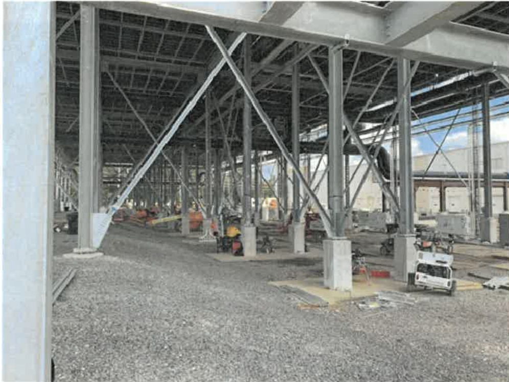
Photo 7-Looking east at ongoing construction under cooling tower structure.
