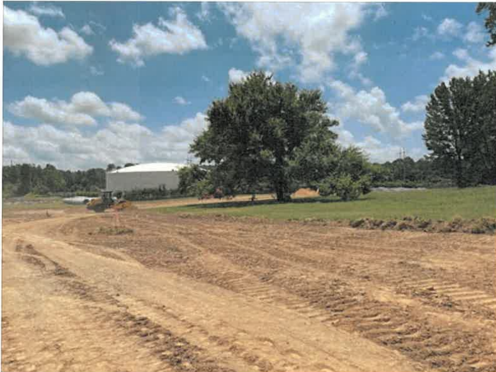
Photo 12-Crews were pushing and compacting this area west of the main section; this area is not included in the disturbed area calculations.
