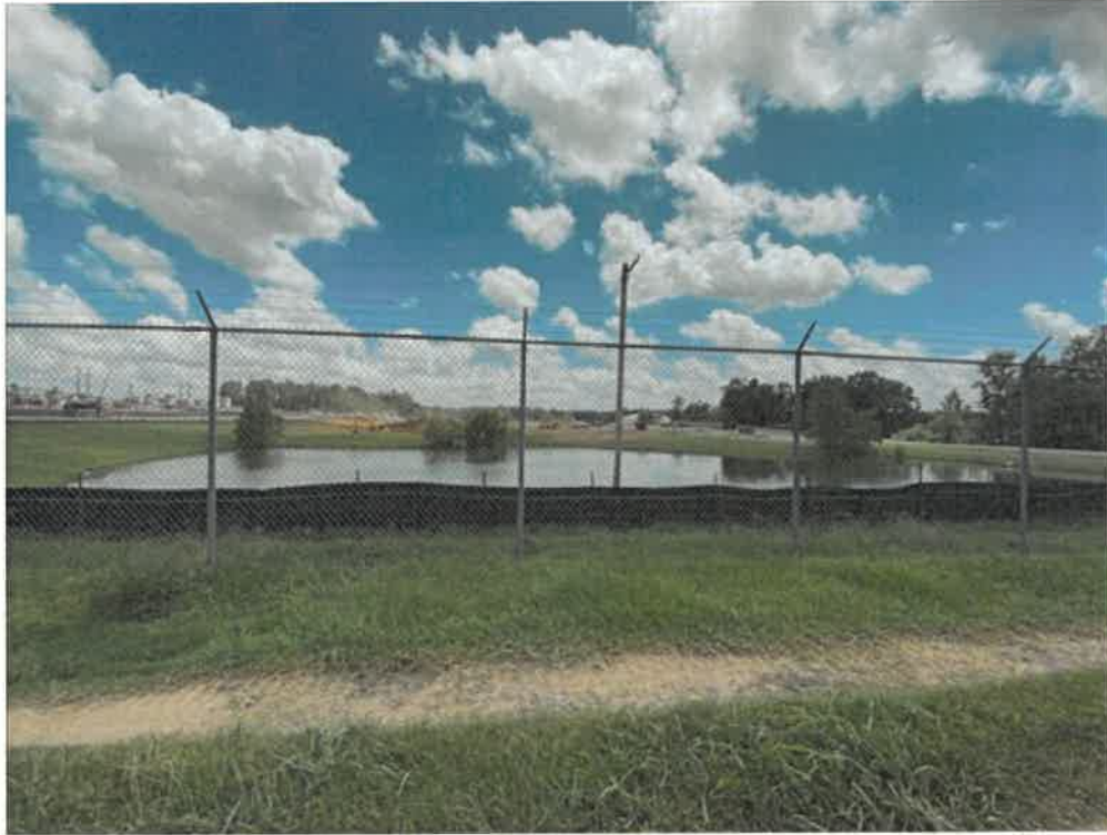
Photo 1-Looking south from Stanton; site has chain link fencing and a run of silt fence around the perimeter. The fencing did not appear to be recently installed. Northernmost pond in foreground.
