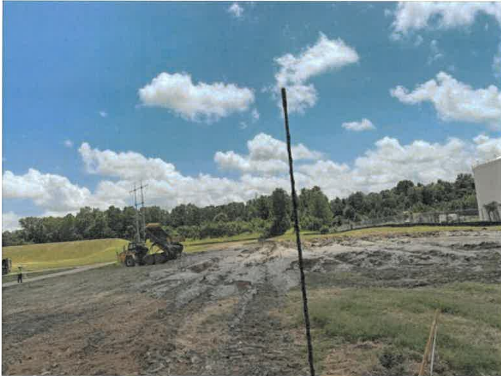
Photo 7-View looking south at pond bottoms being dumped in dewatering area. West end of gun range berm visible in rear left; Horn Lake Sewer tank on right. This is just north/uphill of drainage in Photo 4.
