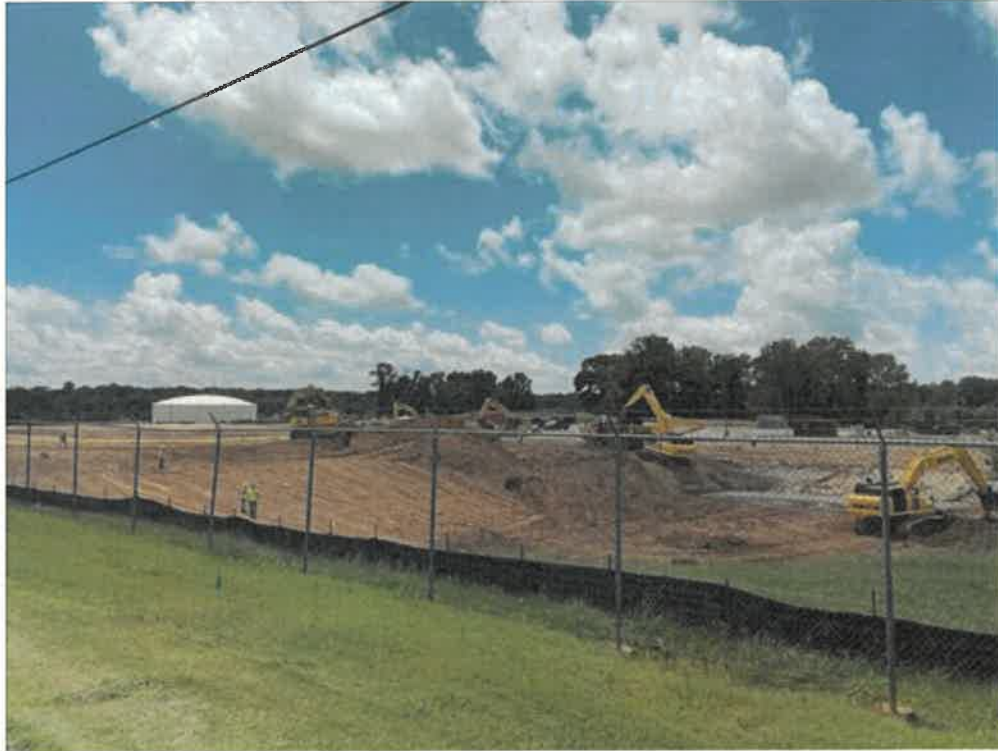
Photo 5-Earthwork going on around small pond.
