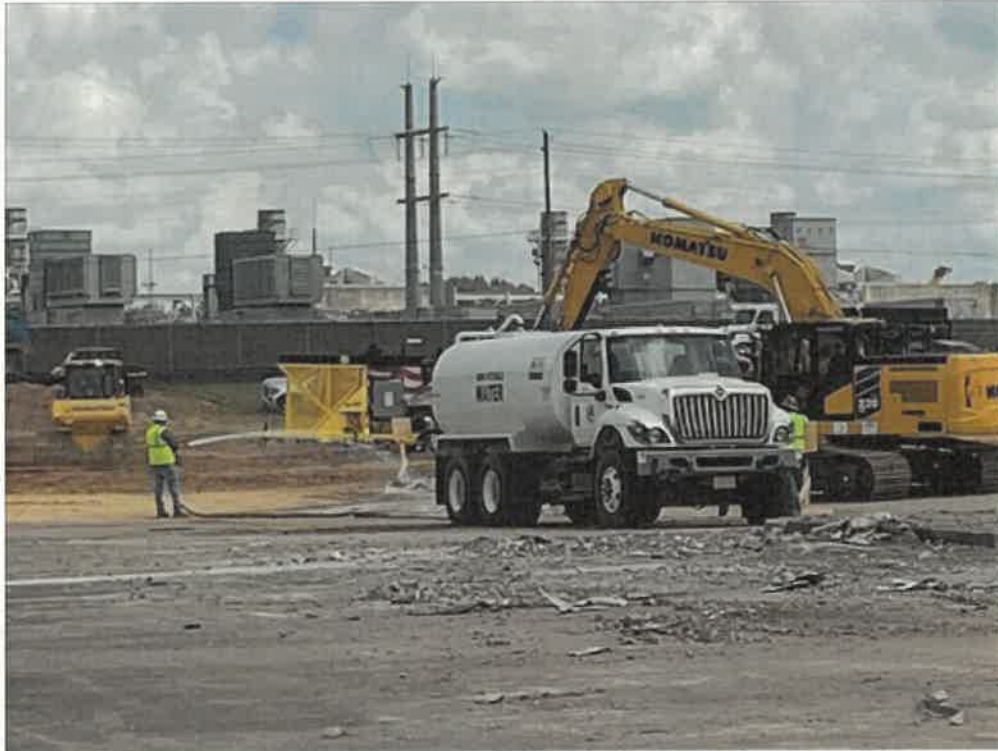
Photo 9-The only water truck observed in use at the site was wetting down concrete for demolition.
