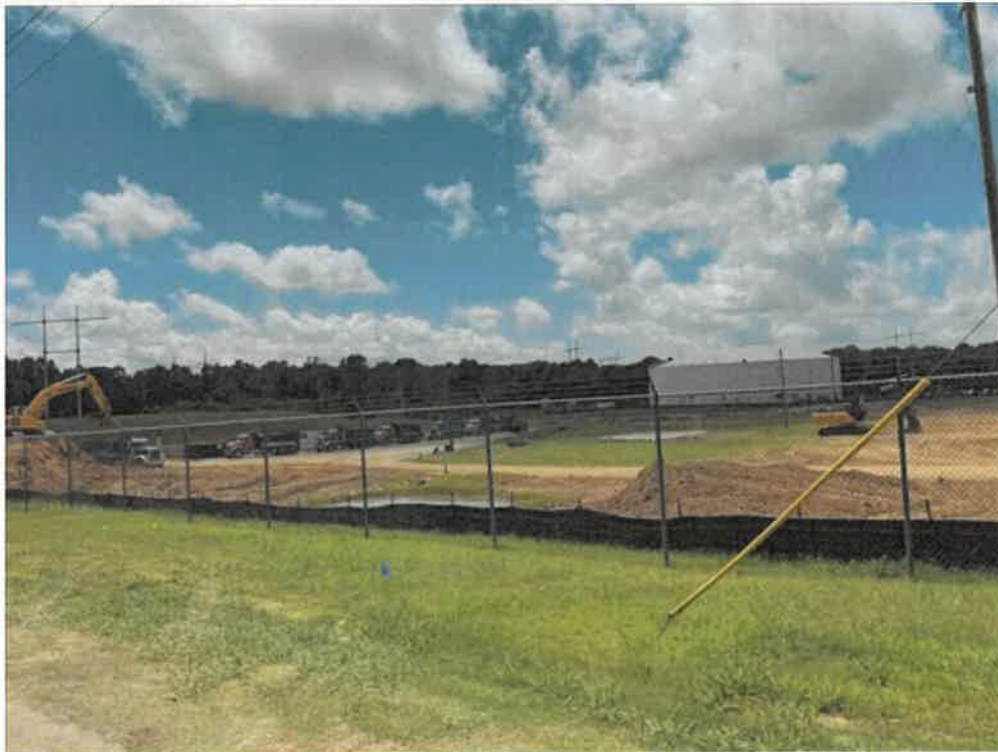
Photo 10-Dump trucks lined up to haul away sections of the gun range berm.
