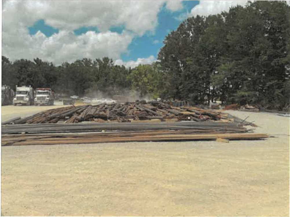
Photo 17-Rebar staging area at Omega lot.
