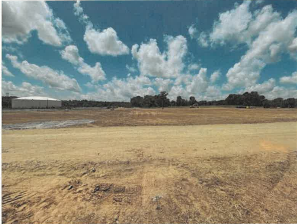
Photo 13-Middle section of the site has been cleared but was not currently being worked.
