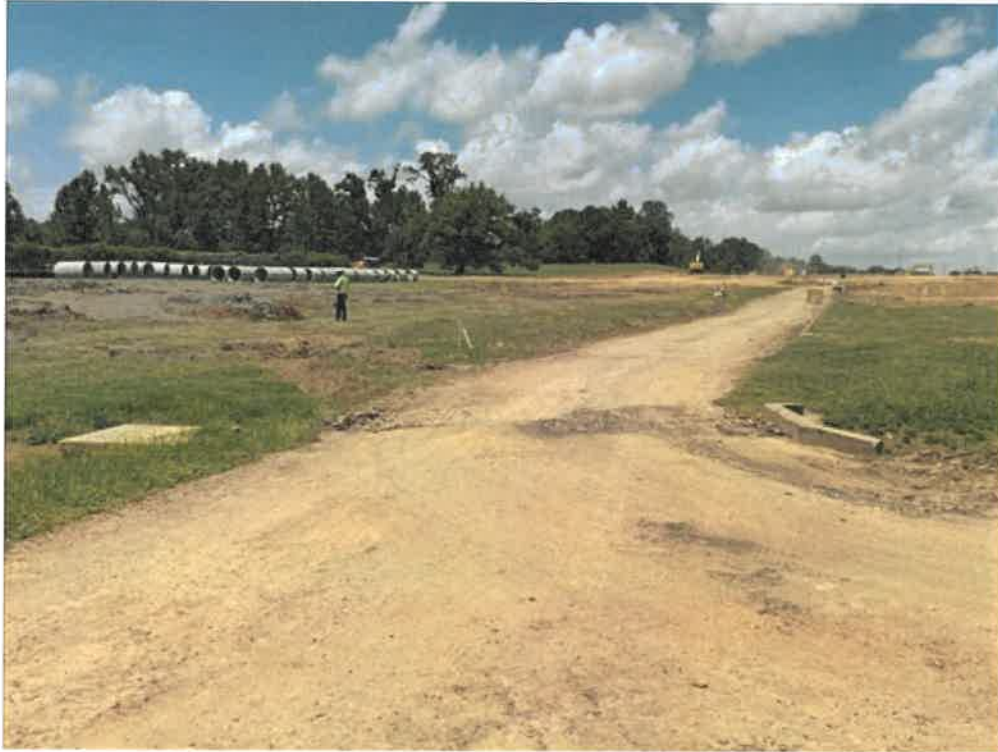
Photo 3-existing tributary across south part of property looking north; no controls along stream or at inlet.
