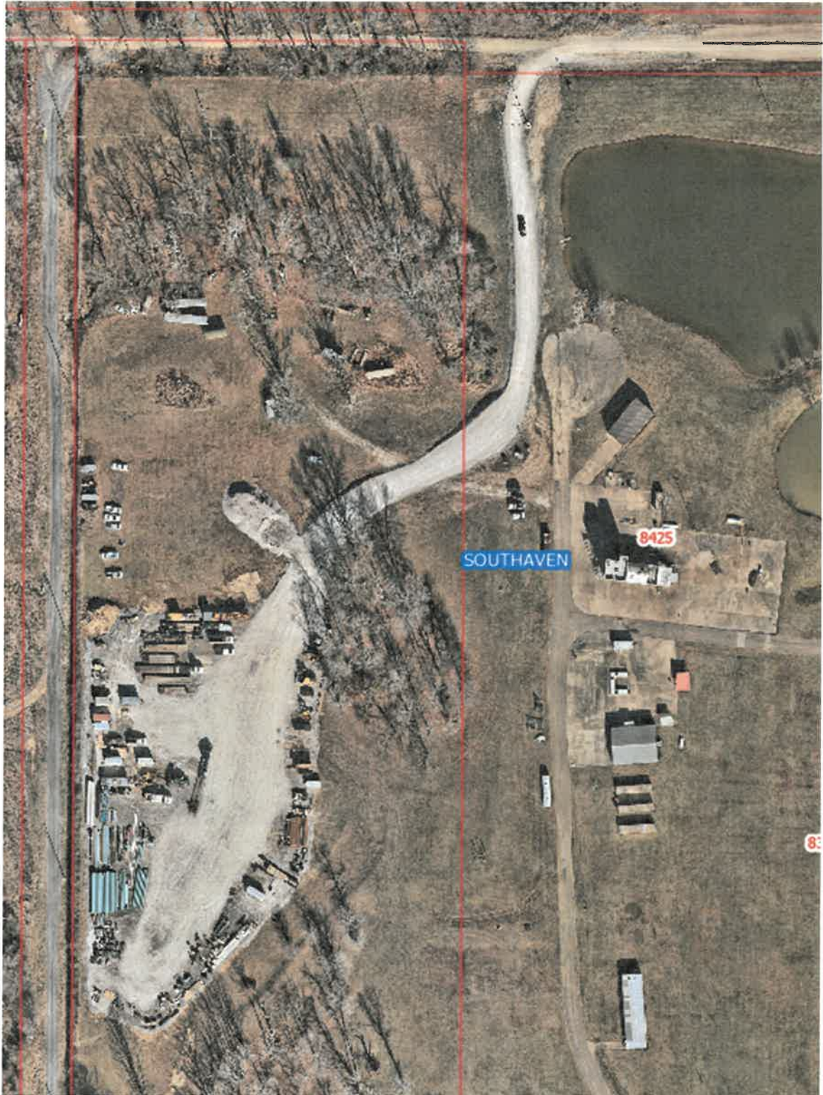
Desoto County January 2026 aerial maps show the area impacted by Omega Foundation Services activities. Note remaining structures on Southaven Municipal Training Facility.
